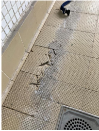
(swimming pool) floor surface
