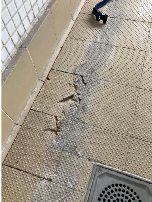
(swimming pool) floor surface
